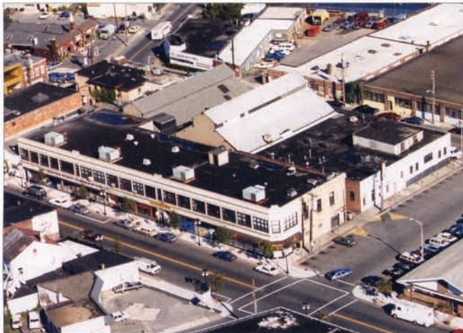
Columbia Northern Corp. entrances plant, Port Chester, New York
