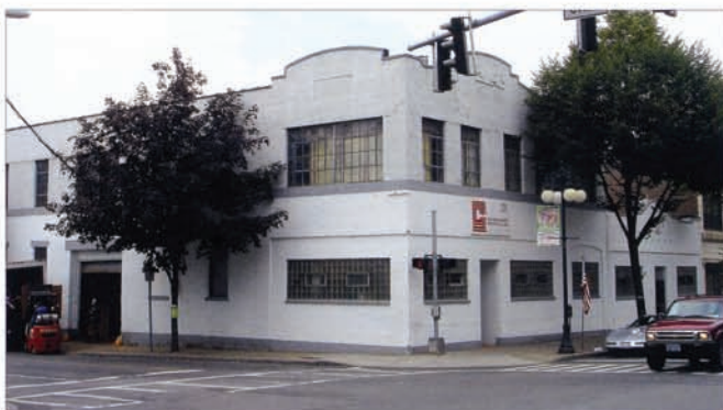
Columbia Elevator Products Co., Inc. corporate headquarters
